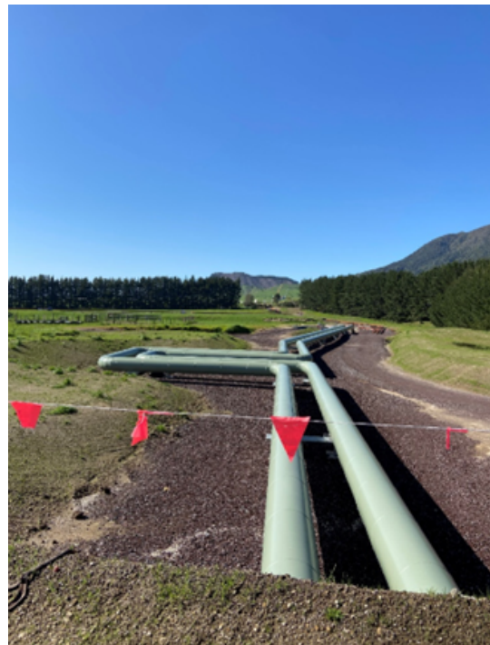
A photo from a Milford trip to the Tauhara Geothermal field. This is piping that takes steam from the drill well to the generation turbine hall to create electricity.
